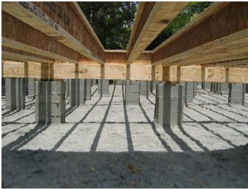
Crawl space with gravel floor
