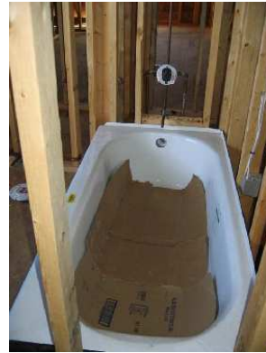
Bath tub(s) set in place
