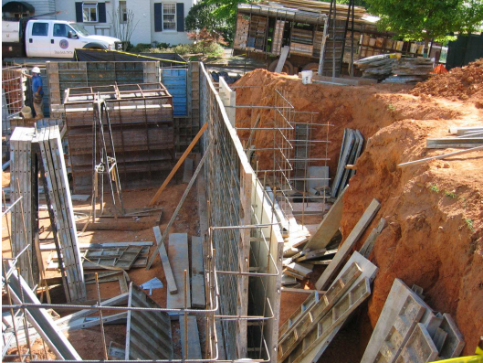
Setting the Forms for pouring
