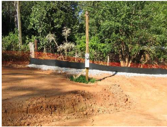
Temporary Electric (Also called "Saw Service")
