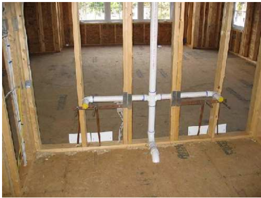
Plumbing "roughed-in" walls
