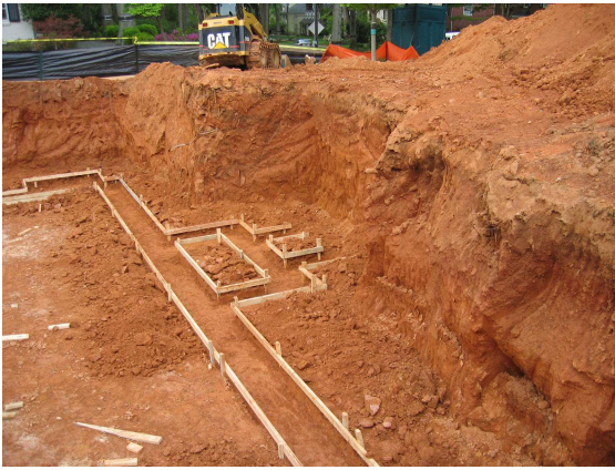
Footing forms set
