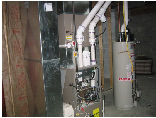
Furnace &amp; water heater "roughed-in"
