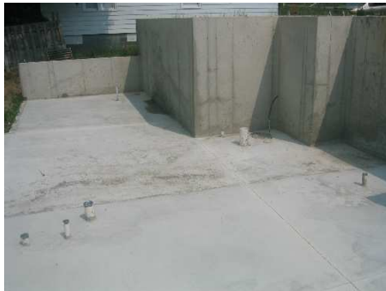
You can see the “rough-in” plumbing
