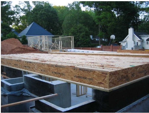
1 st Floor framing
