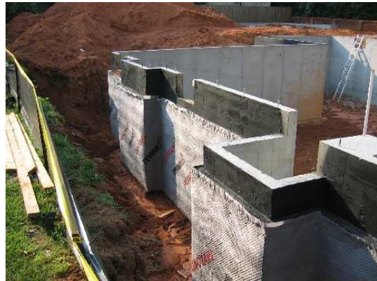
Walls finished & waterproofed
