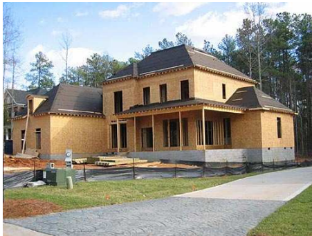
Nearing "dry-in" stage
