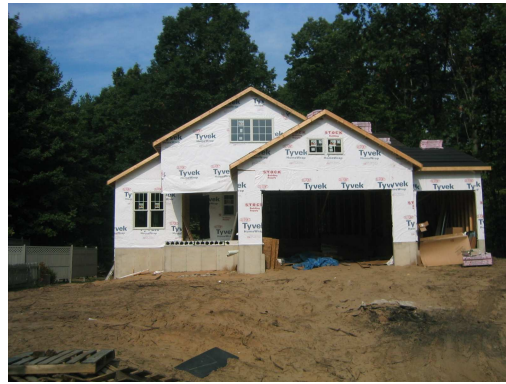
Exterior sheathing &amp; wrap
