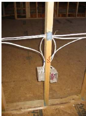
Wiring "roughed-in" walls
