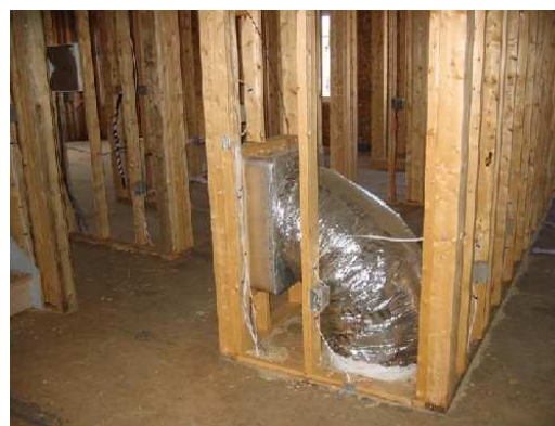
Heat ducts "roughed-in"
