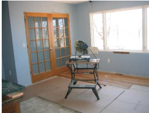
Finished flooring installation
